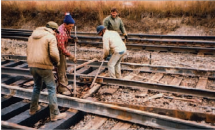
A crew rehabilitates track in the 1980s.
